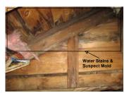
Some of the floor boards have been cut and are now loose. They should be serviced so that the attic floor is
